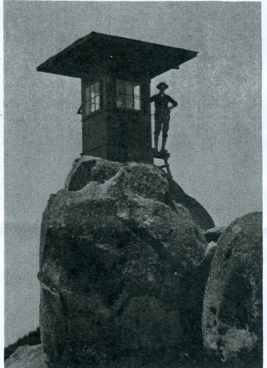
Lyons Peak lookout station, as it appeared around 1918, located in the back country of San Diego County. — John Robinson Collection
